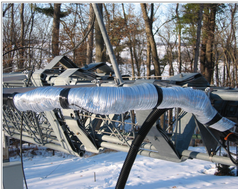
Sheathing over repaired cable bundle. Red Green would be proud.
