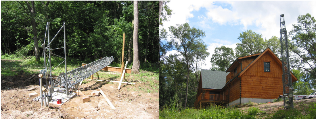
The tower laying over, ready to raise up and the tower raised up to vertical
