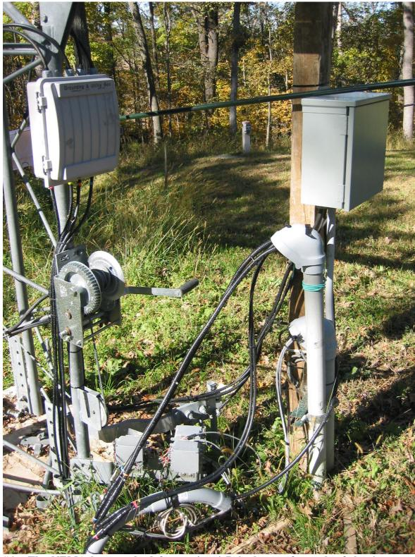
**#6:** The NEMA box on the left contains 4 Polyphasors for each of the 4 runs of coax/Heliax. The box on the right contains the LM470 motor control to raise/lower the tower. The two vertical PVC pipes are split into two: The tall one for the RF/coaxes and the lower one for the 40 control lines. The curved PVC at the bottom runs over to the base of the vertical phased array...about 50'.
