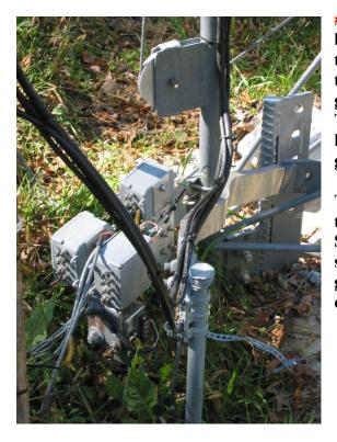
**#5:** This shows the grounding system at the base of the tower. The thick strap runs to that vertical 1" copper pipe. From that there is a #2 copper wire running under ground in a loop to 3 other copper stakes. There is also a #2 copper wire running from here to the house mains and the station ground.
