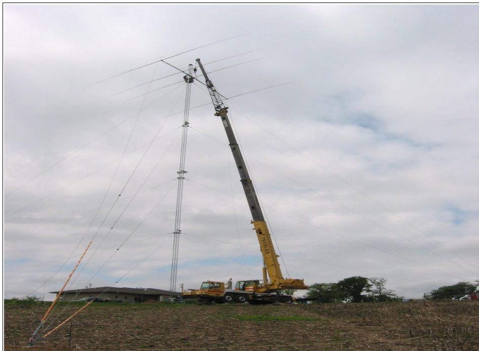
170' crane lifting 4-el 40M beam (50' boom, full-size elements) (M2 manufacturer)
