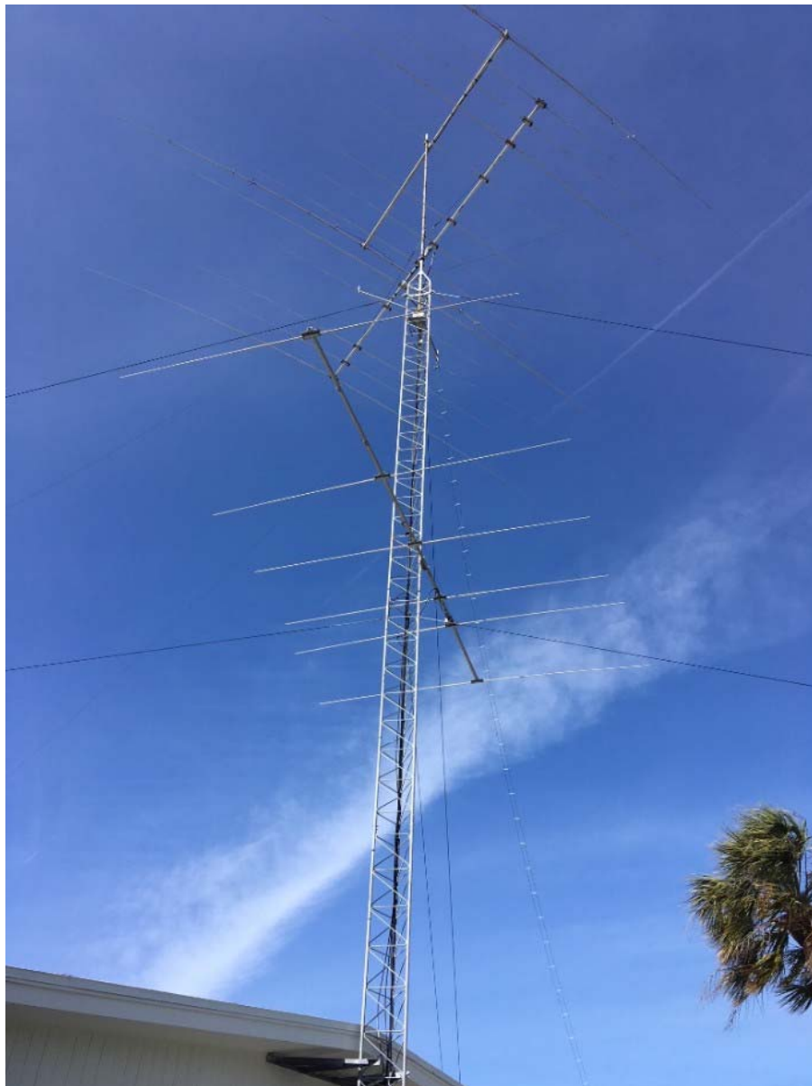
Tri-band antenna at 60'; 2-element 40m beam at 75'. 10m antenna fixed to SE while the ring rotor is down for service.
