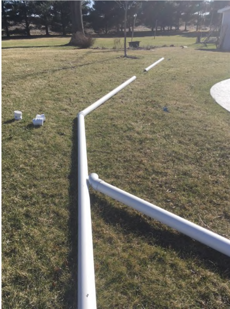
Laying out the conduit - 140' run
