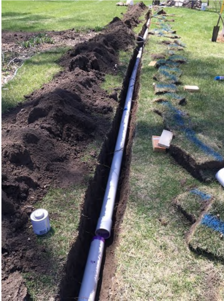
3" PVC going into the ground. Designed with two low spots and set into a gravel bed.
