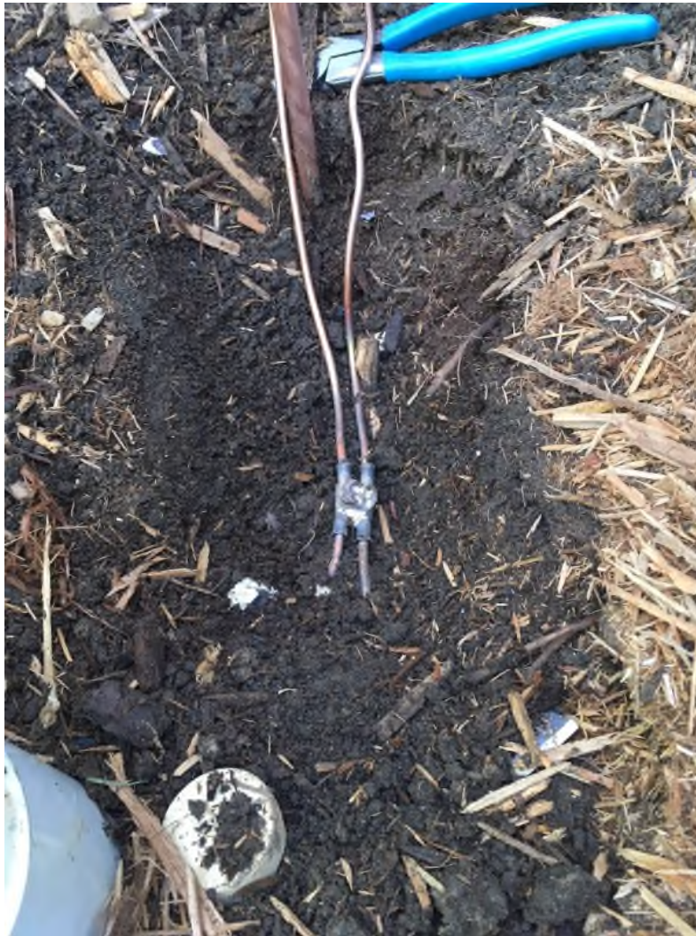
These 4-wire Cadwelds are handy for tying in the lightning panel and the house ground ring
