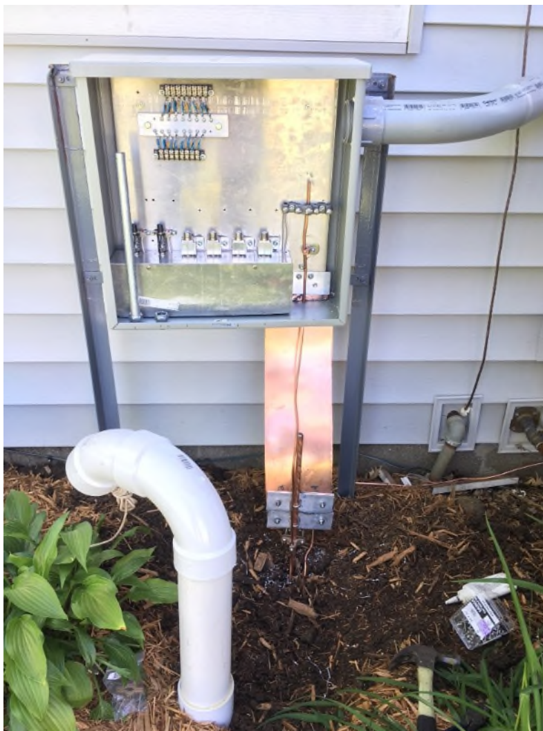
Ground hooked up. 6" copper strap connected to ground rod, backed up by 4ga copper wire.
