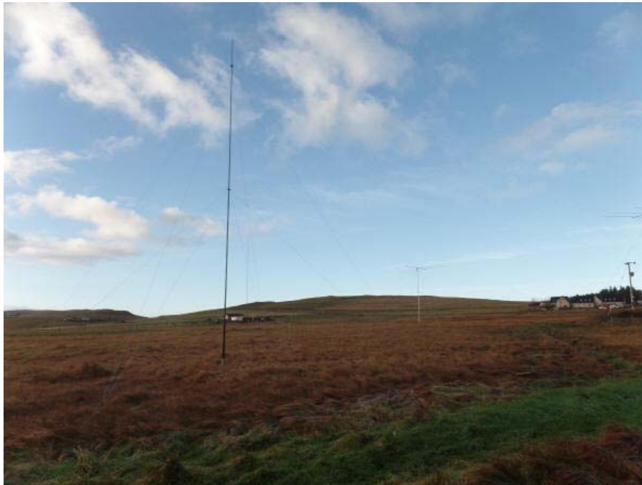
The 16m high top-loaded 80m vertical (with 2 elevated radials)
