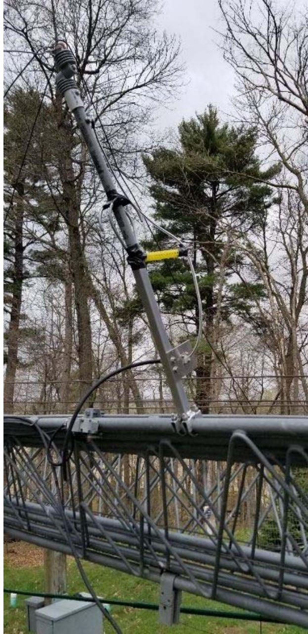
The feed assembly for the reverse feed and the insulators at the end of the PVC for the center fed radials.
