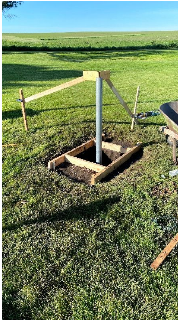
Pipe is held in place before the pour.
